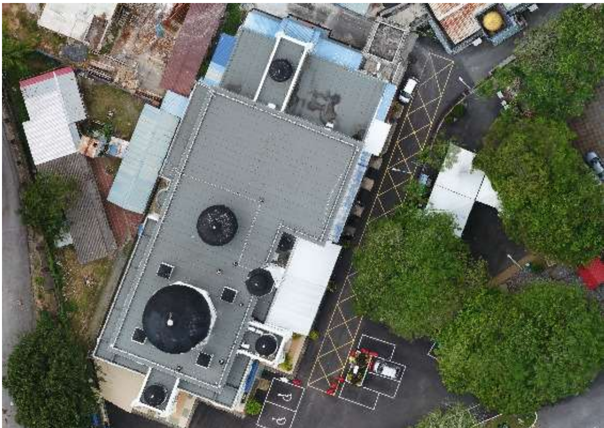
Figure 2.2. An aerial perspective of Alwi Mosque was captured during the data acquisition process.
